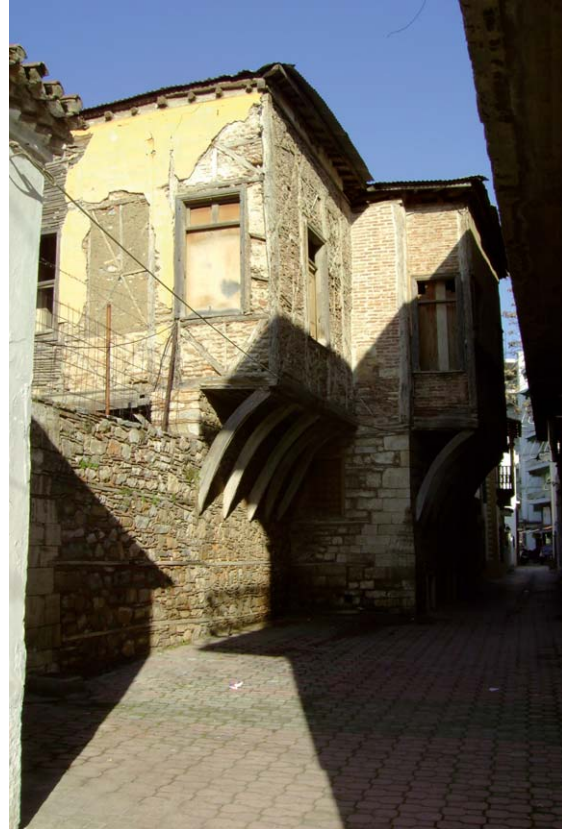
Fig. 15 The Paidon Mansion, view from the southeast
