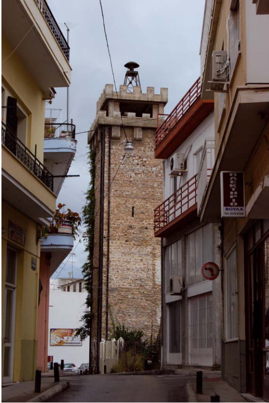
Fig. 14 The Seirina Tower, view from the southeast
